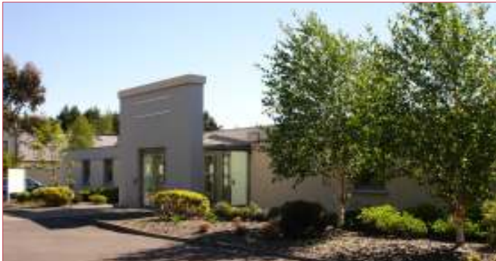
NTDI Building, Tralee
